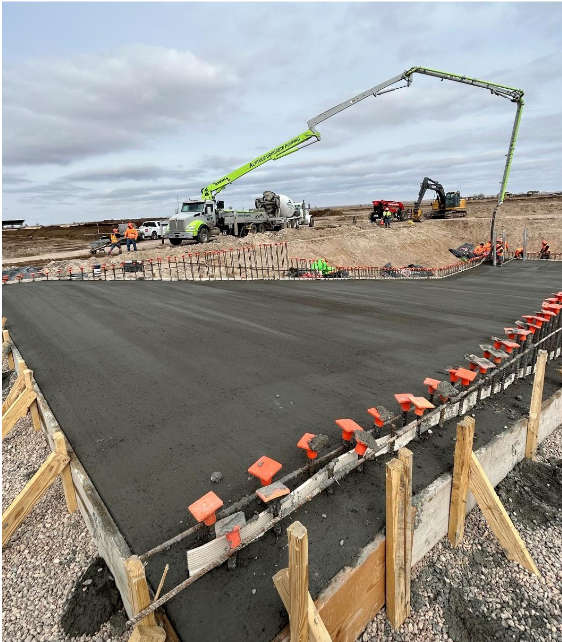
Figure 3. Longs Peak Dairy- fluid retention basin floor.
