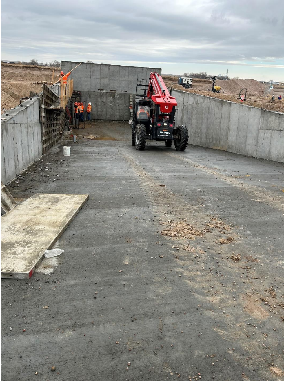
Figure 4. Longs Peak Dairy-fluid retention basin with walls.
